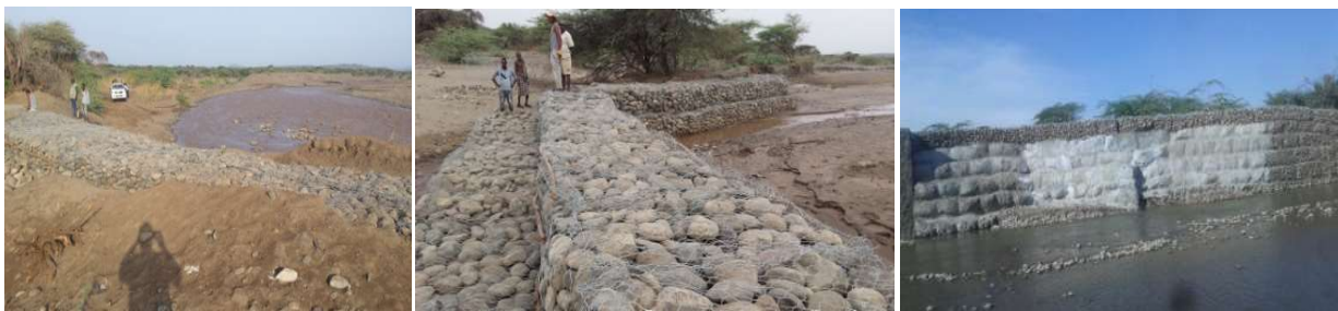
Figure 18: River bank protection work with gabion boxes
