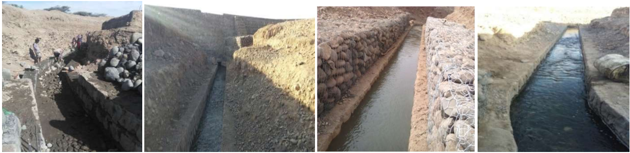
Figure 12: Main canal lining constructed
