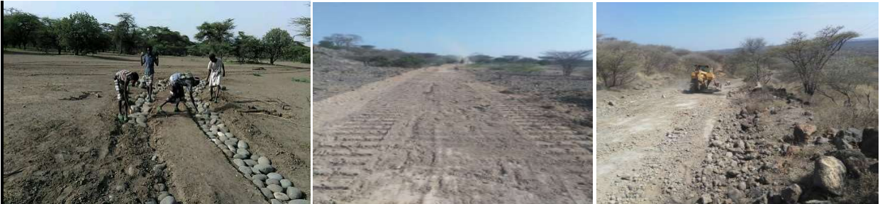
Figure 4: Access road constructed
