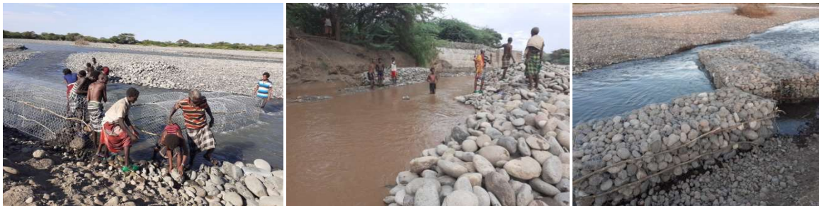
Figure 19: Gabion deflectors constructed
