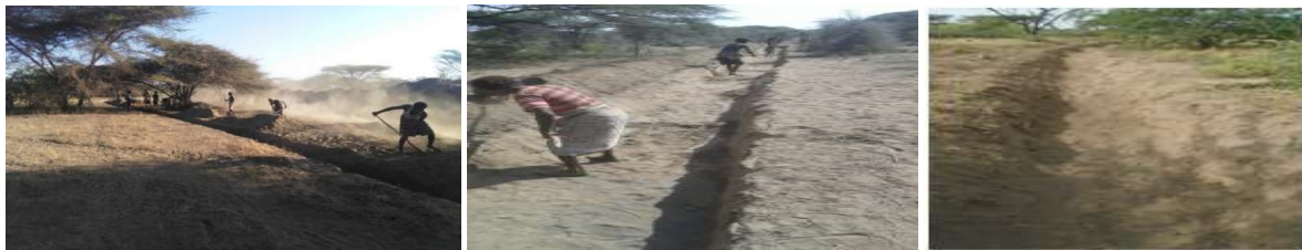
Figure 29: Cut off drain excavated
