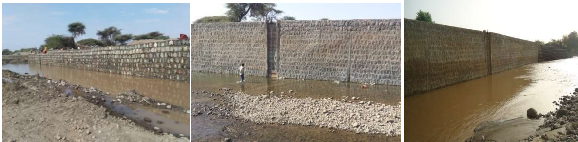
Figure 6: Retaining wall constructed
