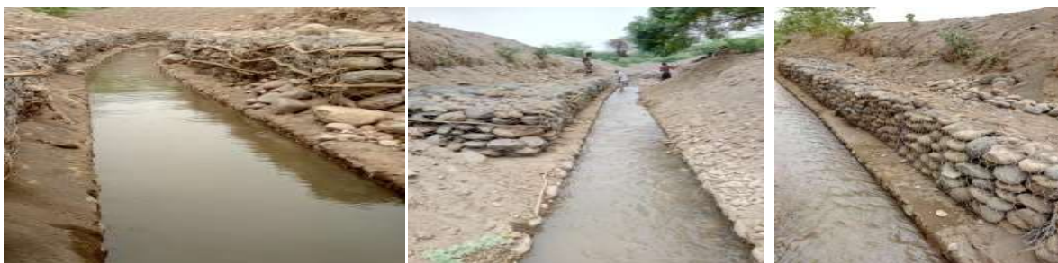
Figure 22: Canal embankment constructed
