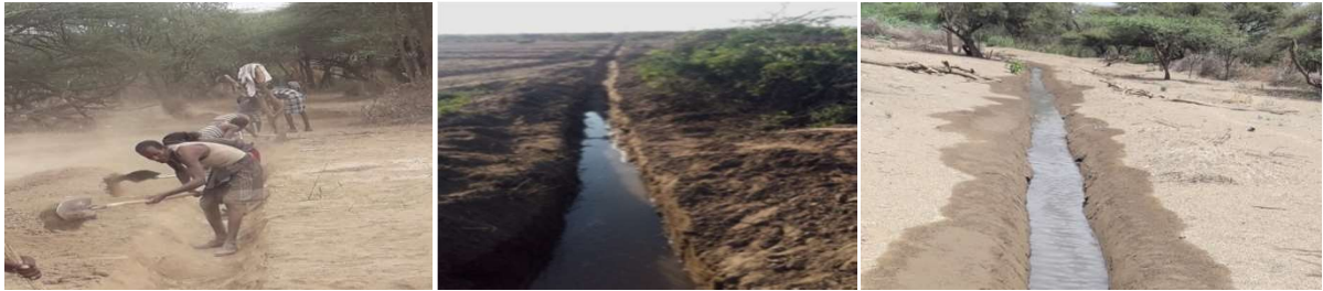
Figure 17: Secondary canal excavated for the new farms
