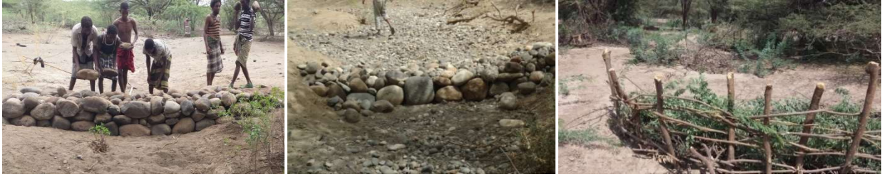
Figure 28: Stone & wooden brush check dams constructed
