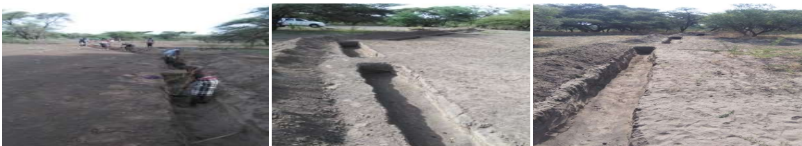
Figure 27: Soil bund excavated
