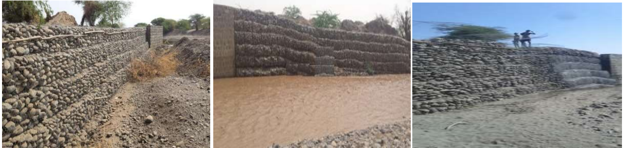
Figure 10: Gabion retaining wall built u/s and d/s of the masonry wall
