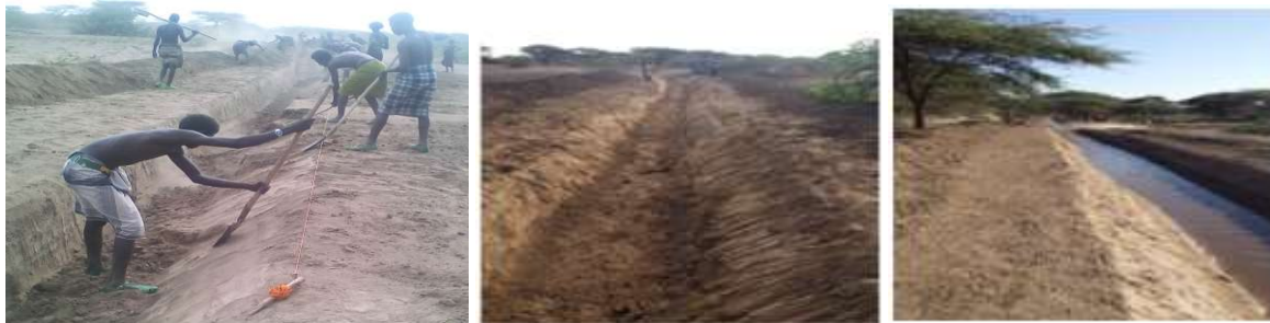
Figure 11: Main canal excavated
