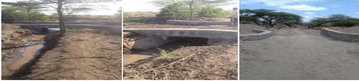
Figure 14: Drainage and road culvert constructed on the canal
