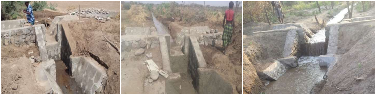
Figure 13: Drop structures constructed on main canal
