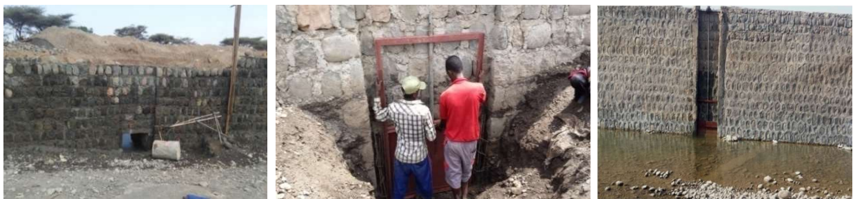
Figure 9: Main gate installed or fixed on the retaining wall
