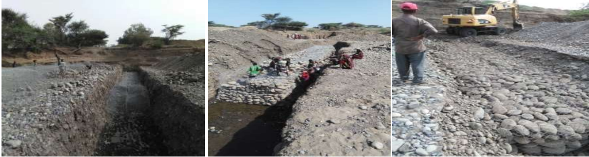
Figure 8: Gabion cutoff wall constructed below the masonry cutoff
