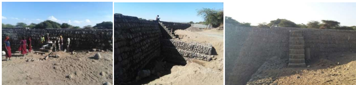
Figure 7: Stair way constructed to walk on top of retaining wall
