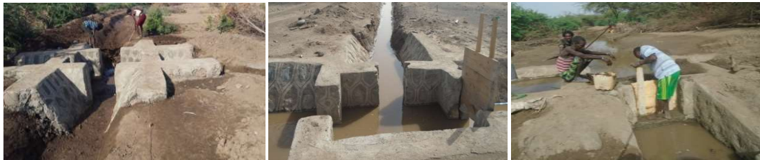
Figure 15: Division box constructed
