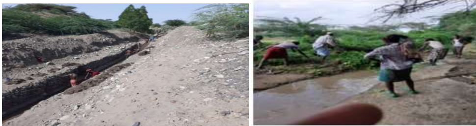
Figure 23: Silt clearing from the main and secondary canal under way
