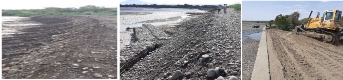
Figure 20: Retaining wall back fill, coffer dam construction and River training work by machine
