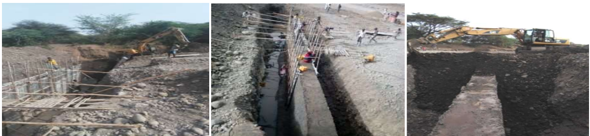
Figure 5: Concrete cutoff wall constructed across the river to intake hole
