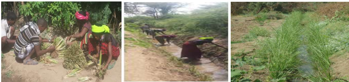
Figure 32: Vetivar slips planted at the canal sides
